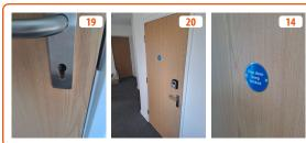
At the time of the assessment, the tenant's door was inspected, and minor damage was observed on the door frame. Additionally, the door handle was found to be loose and may become problematic over time if not addressed. Have the identified issues rectified to ensure the door is suitable and sufficient.
