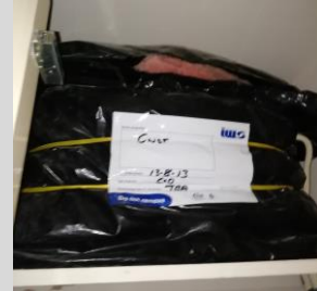
Typical tank in flats 1-12
