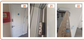
Flat 33 entrance door was sampled at the time of assessment. The door appeared to be of good FD30 timber construction and was fitted with intumescent strips, cold smoke seals, fire rated hinges and a self closing device.
