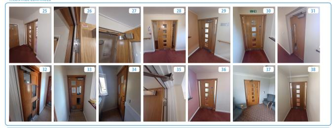
Flat 2 entrance door was sampled at the time of assessment. The door appeared to be of good FD30 timber construction and was fitted with intumescent strips, cold smoke seals, fire rated hinges and a self closing device.
