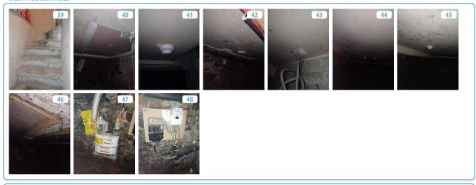
Electrical fuse boards were noted within the means of escape. However, they are of metal construction and, provided they are kept shut, should not pose a significant risk.
