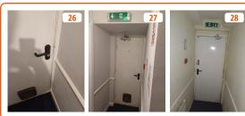
The cross corridor door between the main corridor and fire escape (near to the laundry room) has both a standard lock and a keypad lock fitted. This means that not only are there two methods of opening the door, but also occupants may not be able to walk through from the laundry room side, limiting the number of escape routes on that side of the building. It is recommended that the keypad lock be removed and the door professionally repaired by a qualified contractor.
